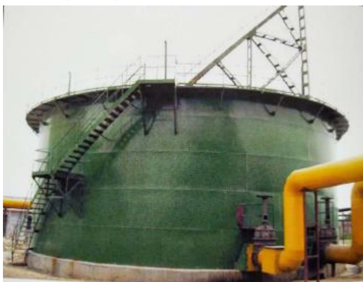
7, Panoramic view of gas station
